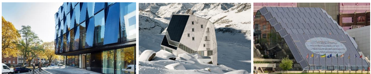
Figure 3 (a) Blauhaus building Germany accordion PV facade (Kaya, 2022), (b) Monte Rosa Hut Switzerland sloped PV facade (Archdaily, 2016), (c) stepped PV facade (Kuby, 2020)
