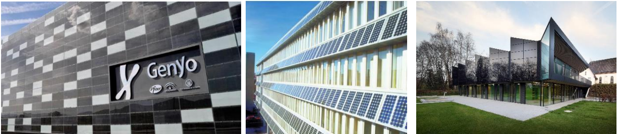
Figure 2 (a) Vertical PV facade, (b) horizontal saw tooth PV facade, (Kaya, 2022) (c) vertical saw tooth PV facade Nursery+E In Marburg/ Germany (Archdaily, 2015)
