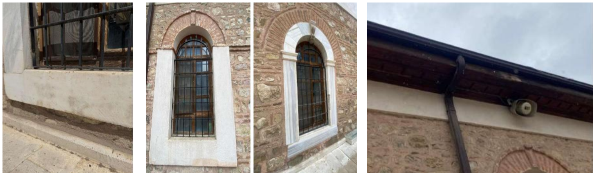
Figure 6. Material deterioration observed on auxiliary elements (Özçelik, Z. S., 2026)
