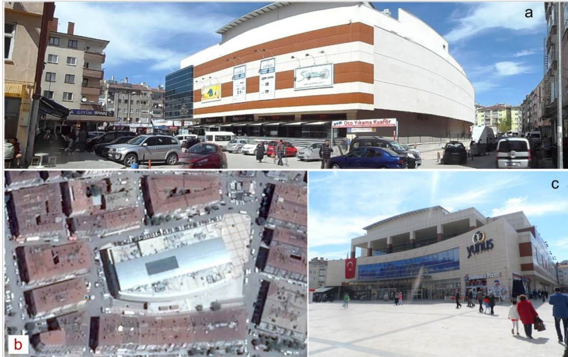
Figure 5. Views of Yunus AVM (a) panoramic, (b) satellite and (c) main entrance façade.
