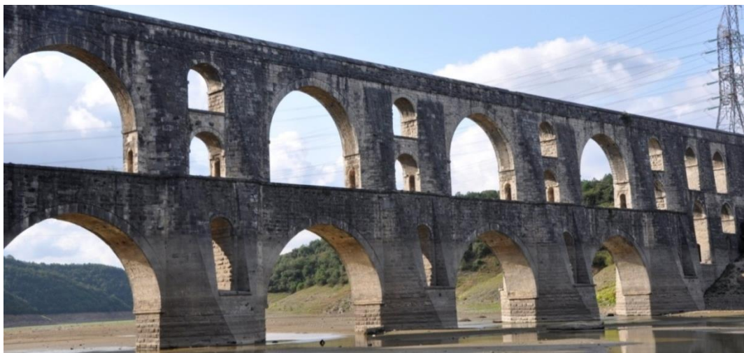
Figure 14. Mağlova Aqueduct lightening belts and buttresses [9]
