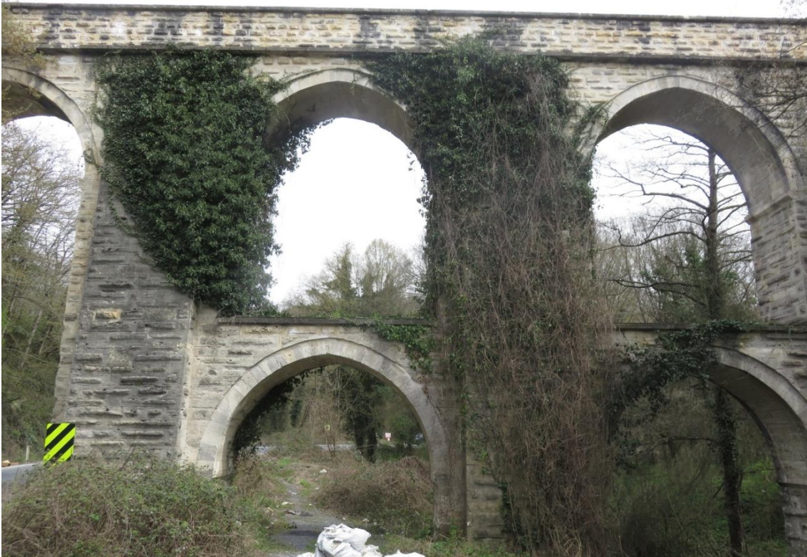
Figure 15. Paşa Kemerli Aqueduct [9]
