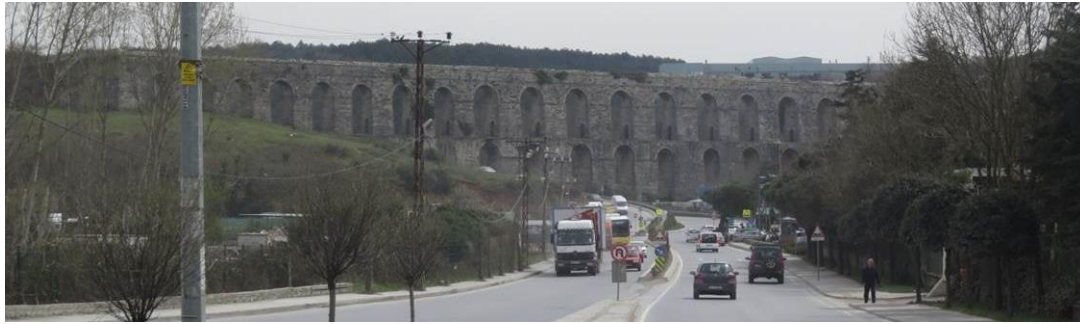
Figure 9. View of Eğri Aqueduct [9]
