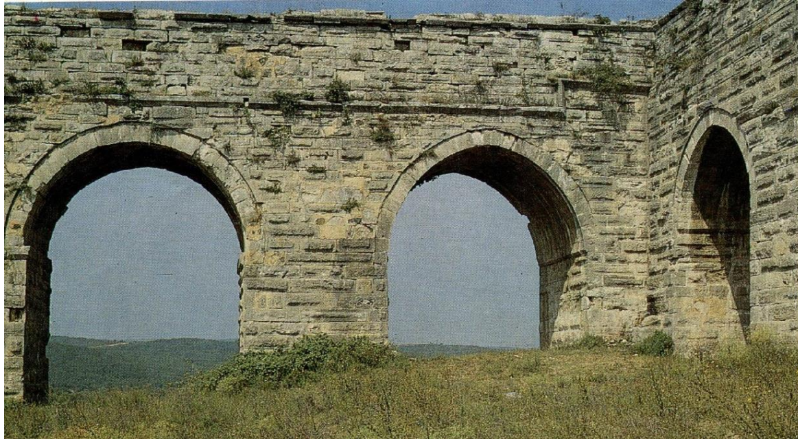
Figure 11. In Eğrikemer, the 14th belt is flat, and the 13th and 12th arches are pointed arches [5].
