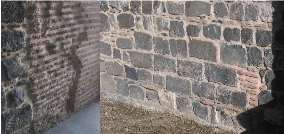
Figure 8. Surface erosion (left) is observed on a brick wall on the western interior of the church and salt accumulations is also observed on the wall of the church south interior facade.
