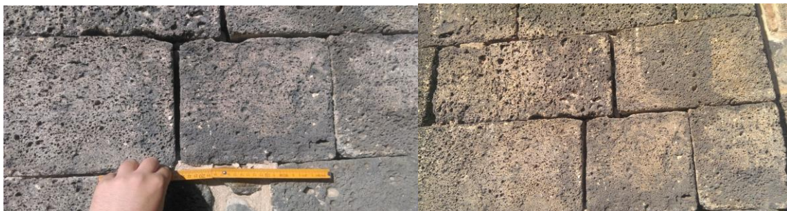
Figure 5. Examples of the type of decomposition related to 10mm joint discharge (left) occurring on the eastern exterior of the church and joint discharge occurring on the south outer facade.
