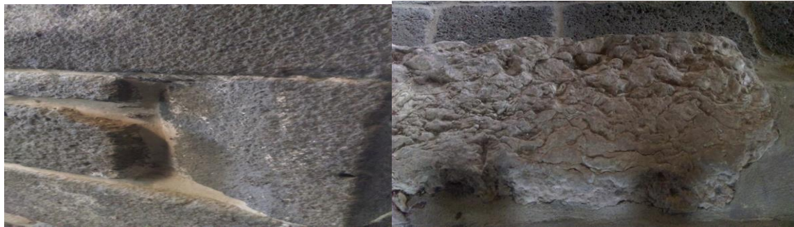
Figure 2. 8 cm abrasion (left) on the wall in the southern interior of Saint George Church (left) and abrasion occurring in the threshold in front of the entrance door
