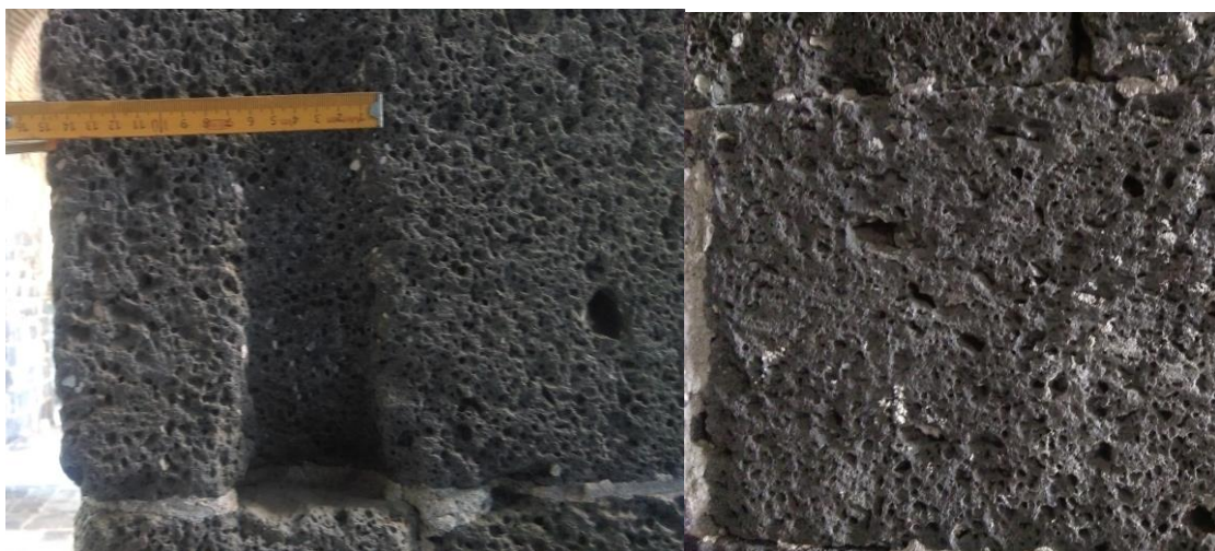
Figure 3. The formation of honeycomb type weathering on the north interior wall of the Saint George Church is seen.
