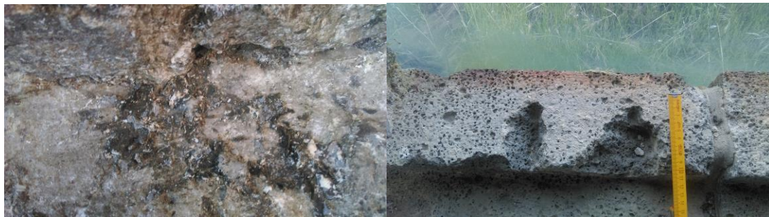
Figure 10. Biodegradation caused by bird droppings on the ground at the south facade of the courtyard of Saint George Church (left). Color change is observed in basalt stones on the church walls (right)
