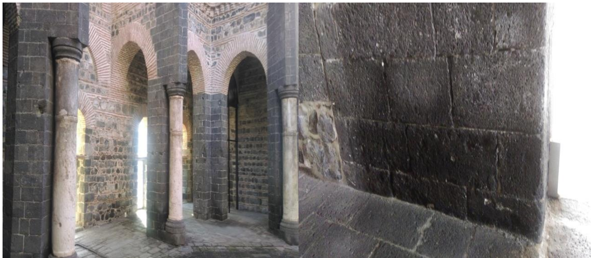
Figure 7. Black layer formation on the columns of Saint George Church (left) and black layer formation under the western wall of the church can be evidently seen.
