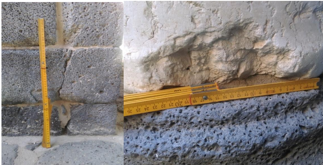
Figure 2. Cracks observed on the wall of the western interior facade of the Saint George Church (left) and a 20 cm fracture occurring in the lower part of the column at the entrance.
