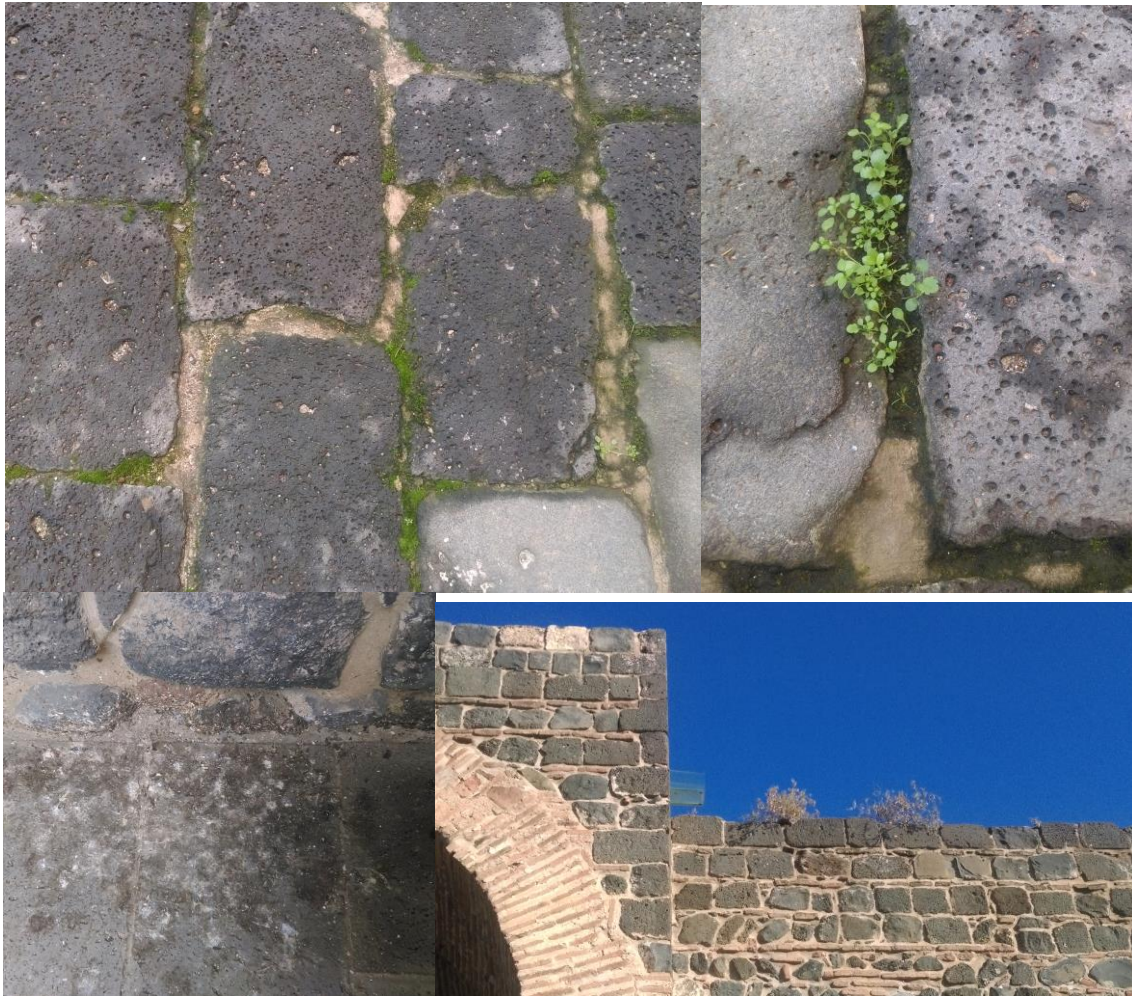
Figure 9. Different types of vegetal colonization are observed on church walls and flooring: Moss development (top-left) between the paving stones on the courtyard floor; herbaceous plants (top-right) formed between the wall joints; herbaceous plant formation on the wall destroyed by algae (bottom-left) occurring in the ground stones in the courtyard of the church.
