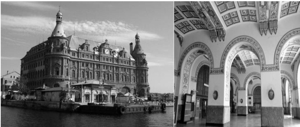
Figure 2. General Views of Haydarpaşa Station.
